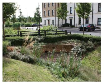
Figure 41: Example of swales check dam integrated with a crossing point elsewhere in uk.
