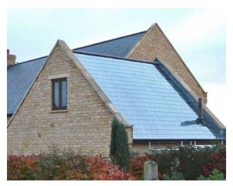
**Figure 55:** Positive example of integrating solar panels at the design stage.
