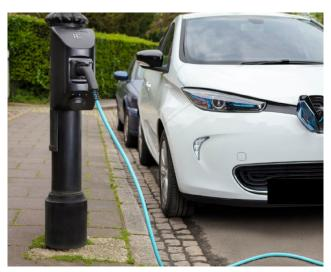
Figure 58: Example of on-street electric vehicle charging points.
