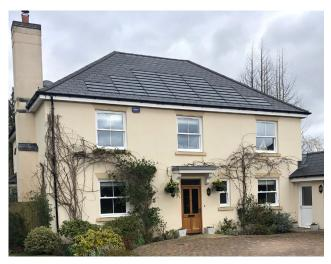
**Figure 54:** Use of shingle-like solar panels on a slate roof, with the design and colour of the solar panels matching those of the adjacent slate tiles.
