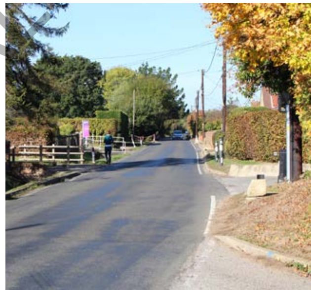
Insufficient provision for pedestrians on Lower Road
